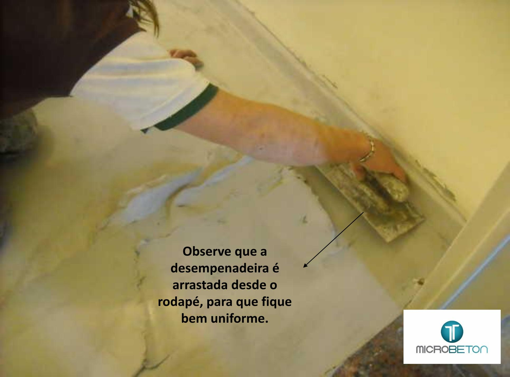
A person wearing a white shirt and a green wristband is using a trowel to finish a concrete floor. The floor is light-colored and has some darker patches. The person is standing on the floor, and their hand is visible holding the trowel. The background shows a white wall and a baseboard.
