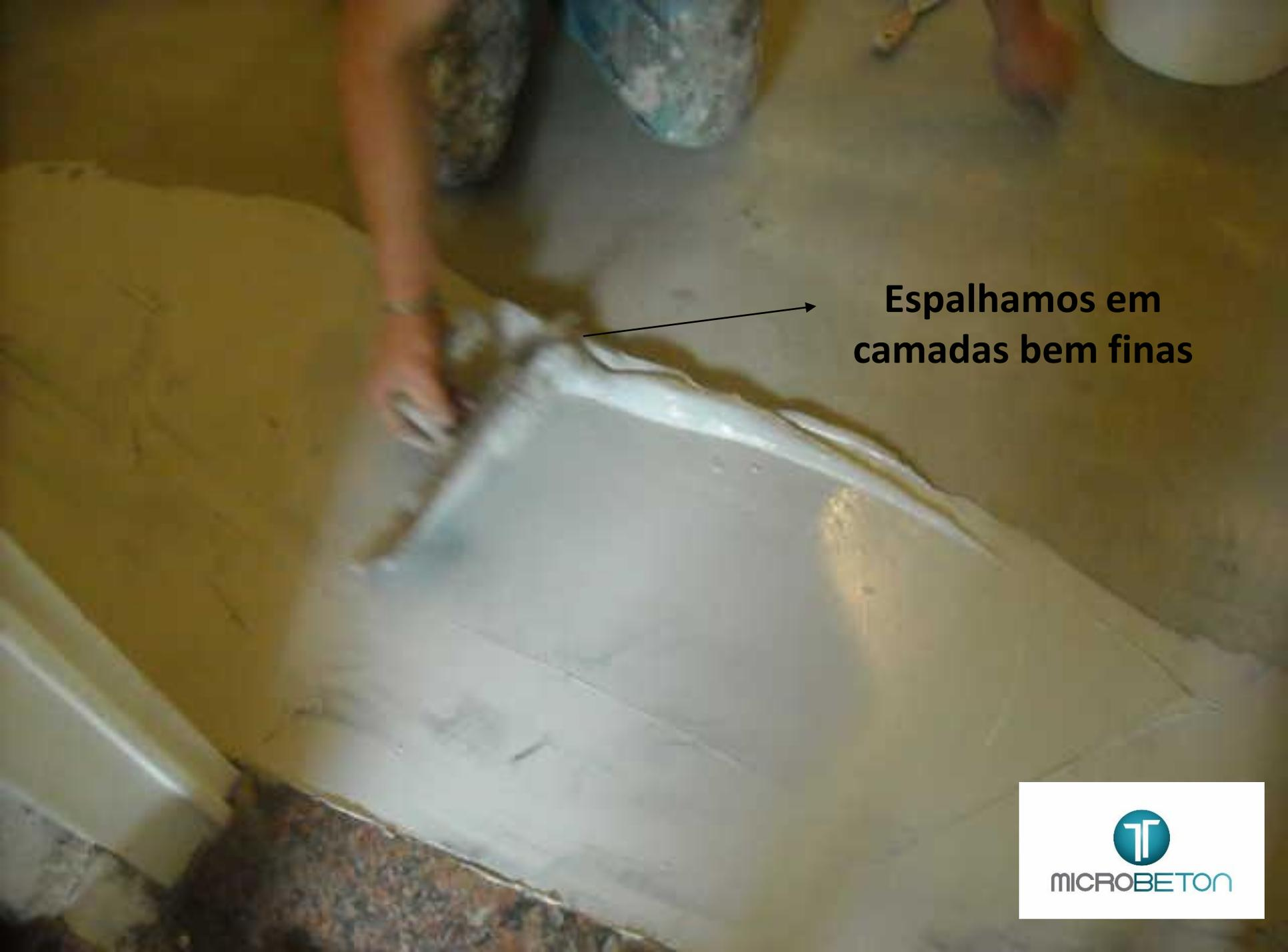
A person is kneeling on a concrete floor, applying a white, paste-like material in thin, overlapping layers. The person's hands and legs are visible, and they are wearing patterned clothing and blue sneakers. The floor is light-colored and shows some signs of wear. The white material is being spread across a rectangular area. An arrow points from the text to the material being applied.
