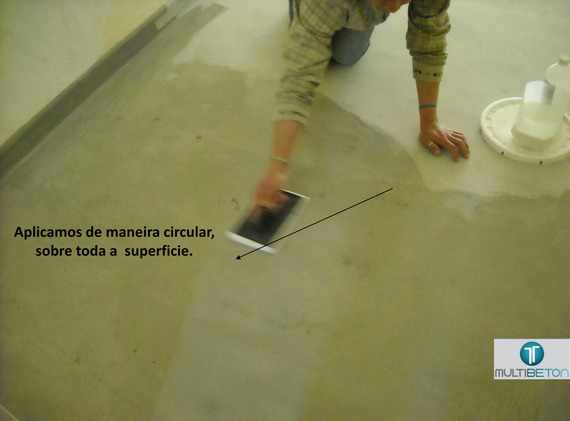
A person wearing a plaid shirt and blue pants is kneeling on a light-colored concrete floor. They are using a brush to apply a dark liquid product in a circular pattern. To the right, there is a white plastic bucket with a white cap and a white bottle. The floor shows some darker, wet areas where the product has been applied.
